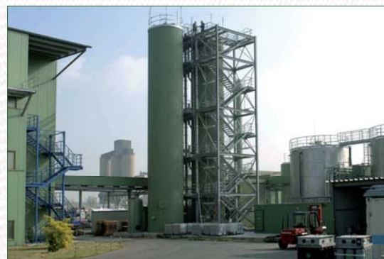
Figure 3.- Full scale installation at a biodiesel production site
