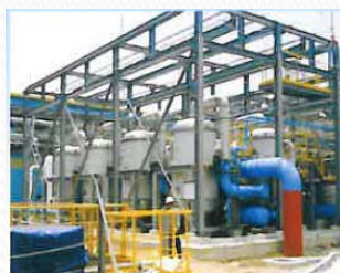
1 train of 8 modules (Ø 1600 mm - H 3500 mm)
